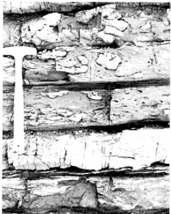
FIG. 10. Beds of disrupted sandstone and mudstone interbedded with thin undisrupted beds of mudstone. This soft-sediment disruption of the stratification is indicative of repeated surface sliding of unstable material of facies 4. Location at 471 m in Section C, figure 4.
