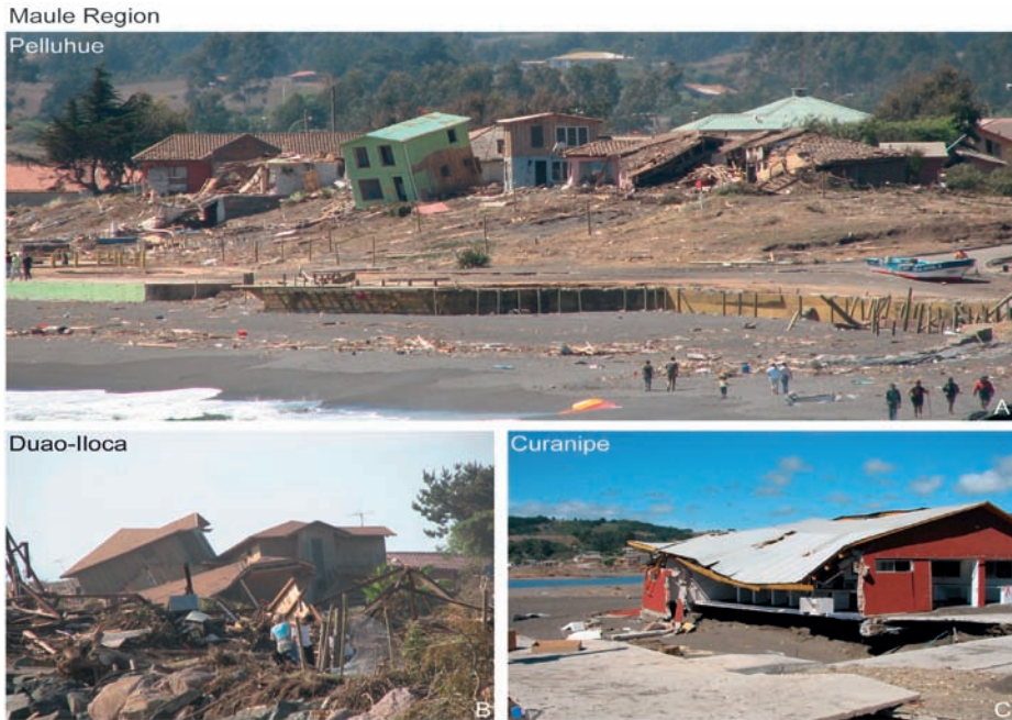
FIG. 9. Photographs evidencing strong tsunami impact along the coast of Maule Region. A. , B. Littoral area affected by tsunami inundation at Pelluhue and Duao-Iloca, respectively; C. Tsunami impact at Curanipe, evidencing a strong effect of erosion processes on foundations of coastal infrastructure.
