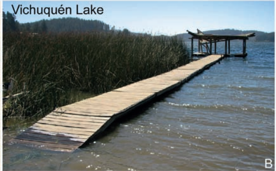
FIG. 6. A. Land subsidence evidenced by flooded fluvial terraces at the Llico River, and B. by partially submerged peers along the margin of the Vichuquén Lake, close to the coast.
